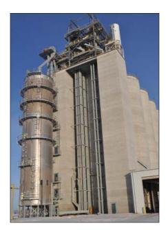
The Hamberg terminal operates five bucket elevators seen in alcove and a 7,000-bph Zimmerman tower dryer at left.
