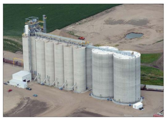
The Hamberg, LLC 2013 rail terminal in Hamberg, ND is a joint venture between CHS and Fessenden Coop Association. One-million-bushel slipform concrete annex at right was completed at the beginning of 2015. Aerial photo courtesy of Vigen Construction Inc.
