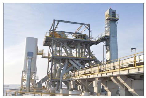
Twin 20,000-bph receiving legs and eight-hole rotary distributors feed grain into overhead 20,000-bph drag conveyors for transport to storage.
